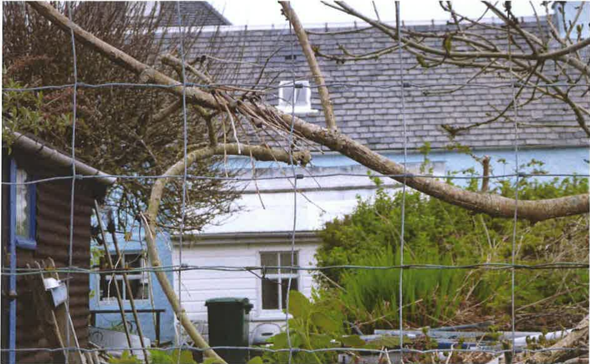
Figure 13 : Timber Clad, Metal Roofed extension (Victoria St)
