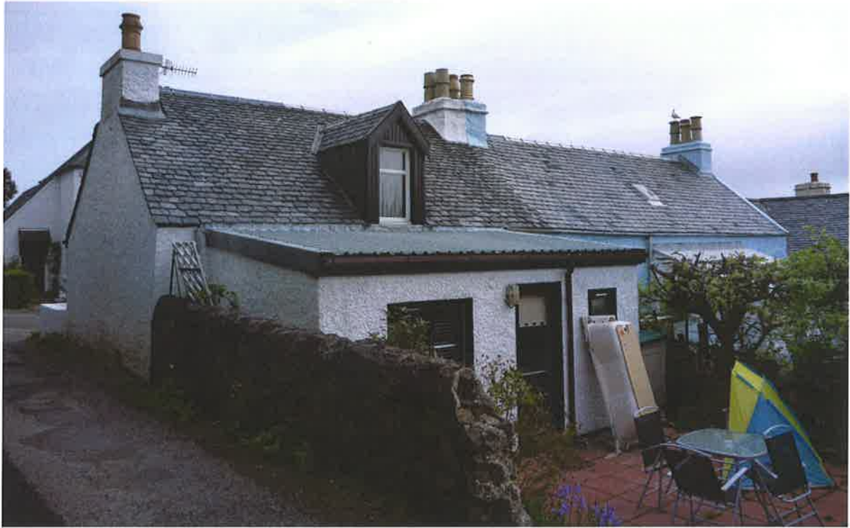
Figure 12 : Profiled metal roof (Victoria St)
