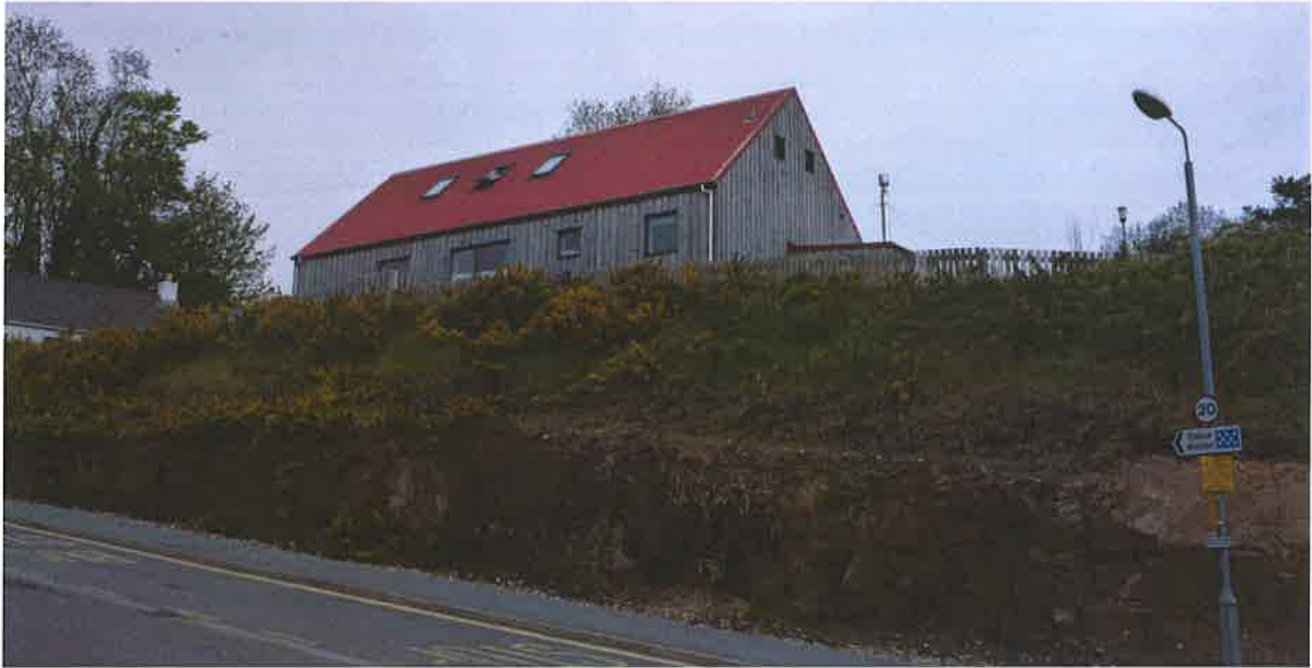
Figure 8 : New Primary School Building on periphery of Conservation Area
