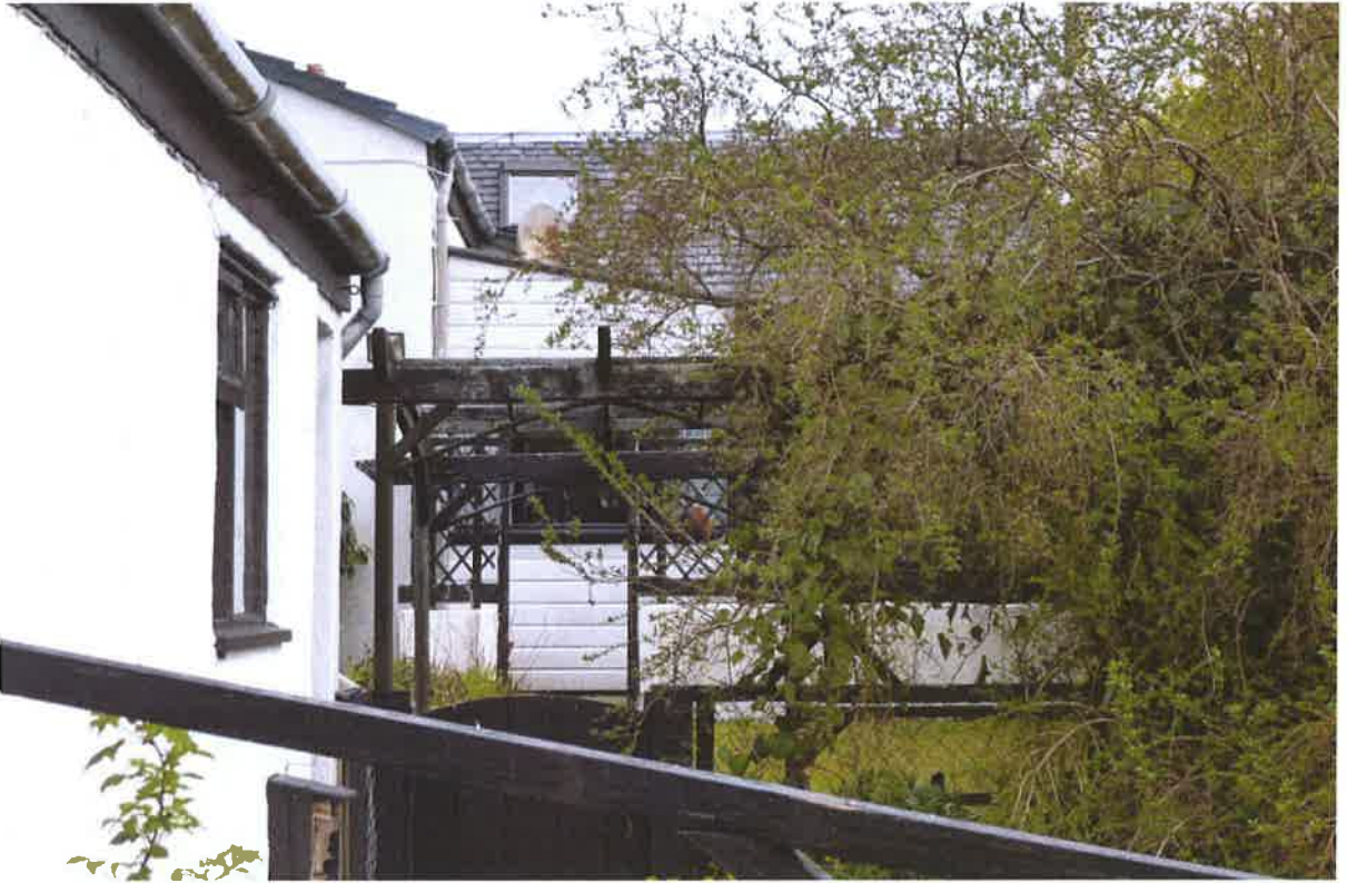
Figure 15 : Timber Clad, Felt Roof Extension (Victoria St)
