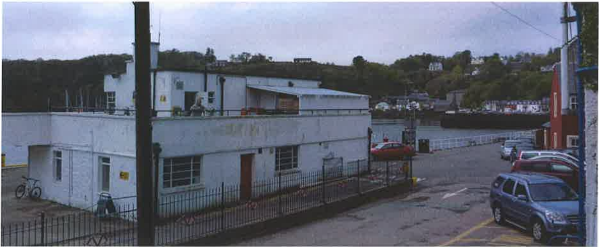
Figure 3: Metal Sheet roof and wall materials on extension to Listed Building on Main Street
