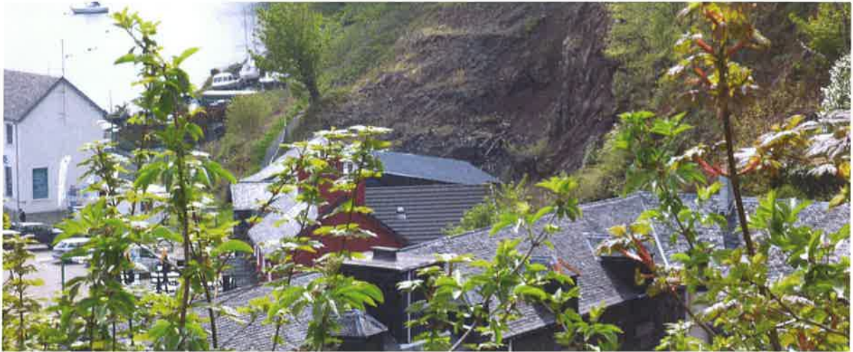
Figure 1 : Macgochans Pub, Tobermory - Original fishermans cottage extended (significantly) with a large profiled sheet roof and timber cladding to the rear of the building
