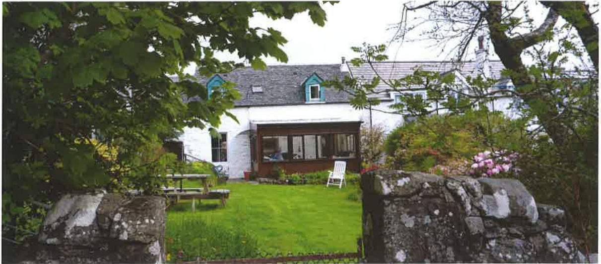
Figure 16 : Timber Clad, Plastic Roof (Albert St)
