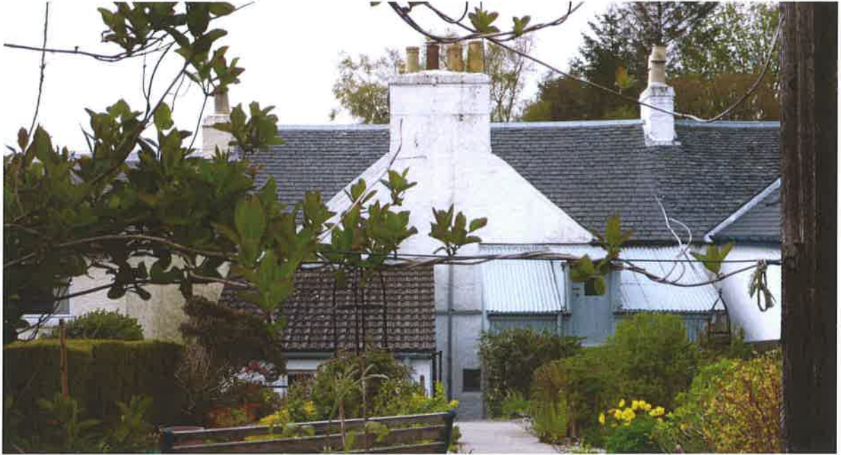
Figure 14 : Corrugated Metal Extension (Albert St)
