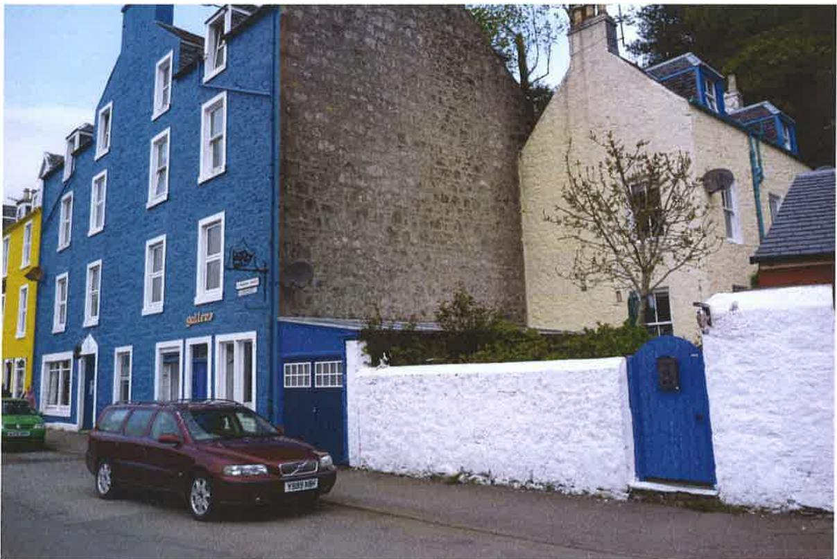
Figure 2: Profiled sheet roof and painted Timber cladding on main street
