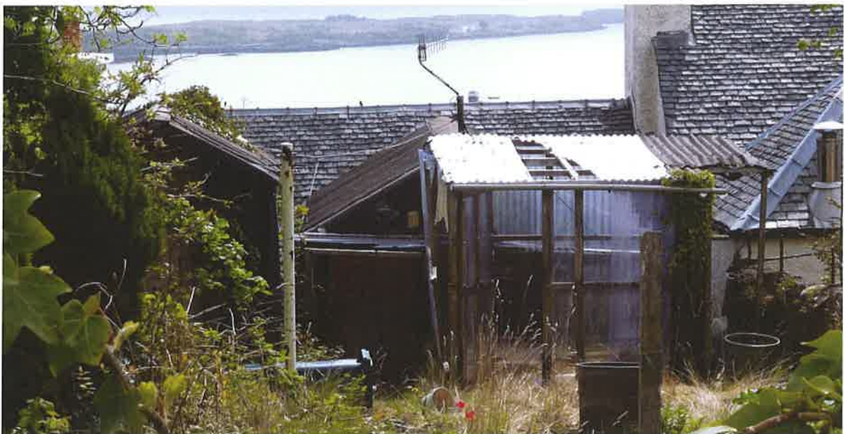
Figure 23 : Corrugated Materials used for extension (Argyll Terrace)
