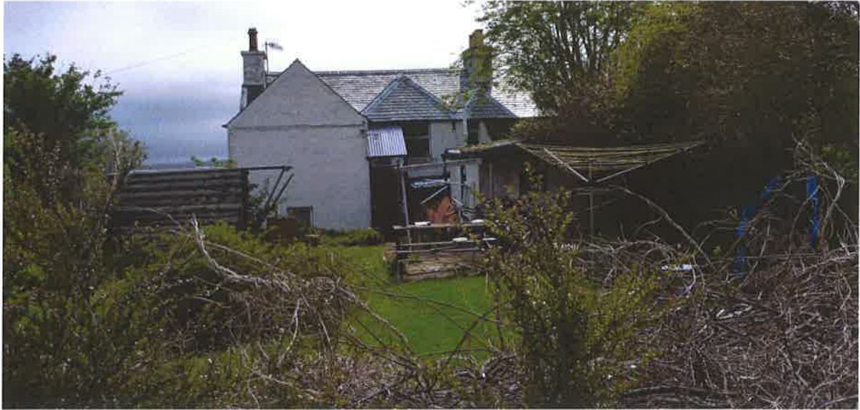
Figure 18 : Various materials used (breadalbane St)
